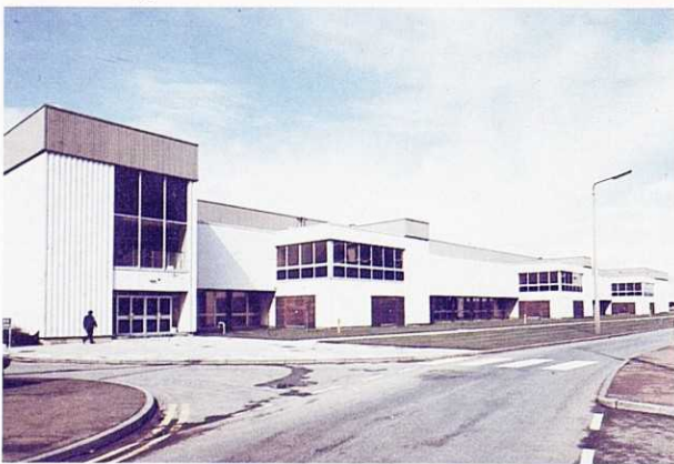
▲ Top: Chemical production—computer control room at Cramlington, Northumberland
